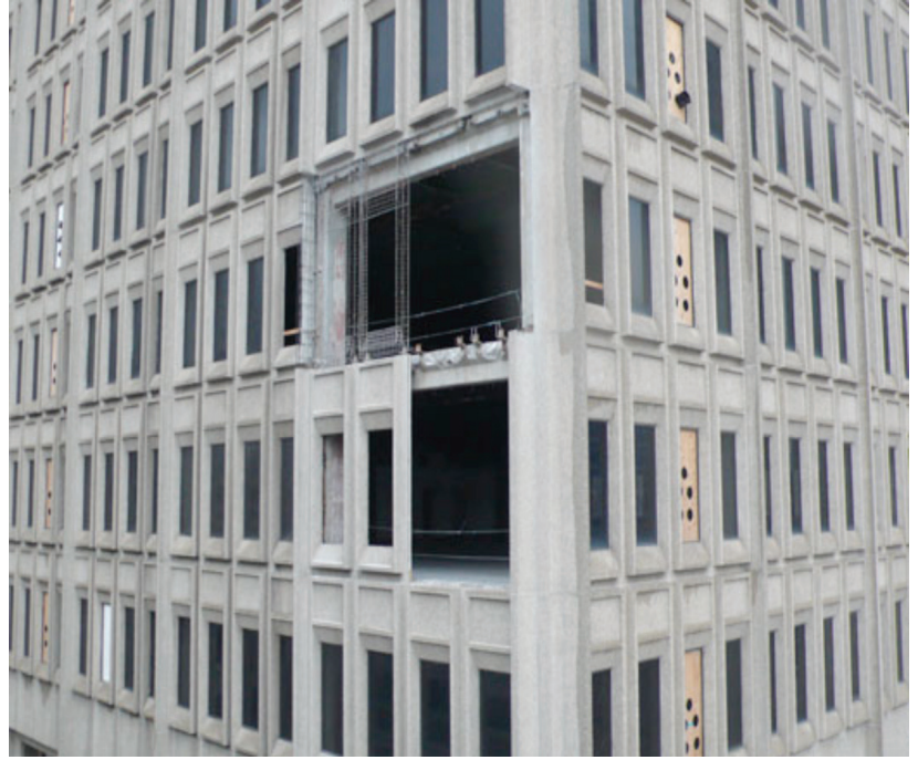
Removal of exterior facade underway
