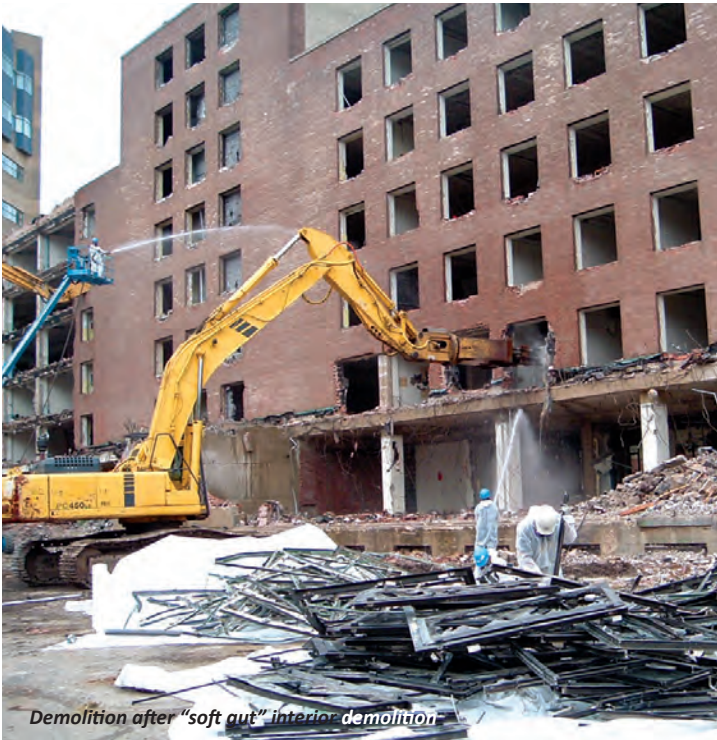
Structural demolition with LVI's high reach equipment
