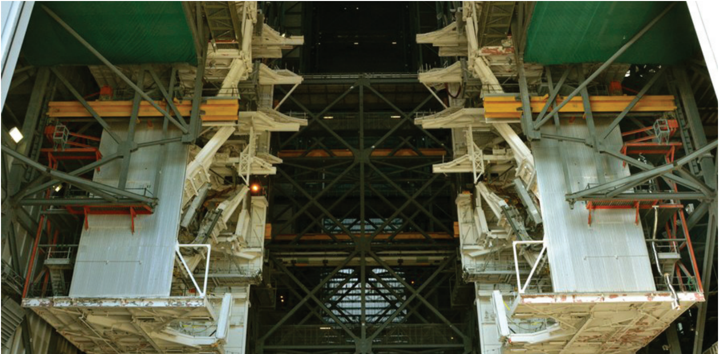
All the white shuttle work platforms shown were removed. Other, more modular structures will be put in their place to accommodate a variety of launch vehicles Photo Credits: Julian Leek / Blue Sawtooth Studio
