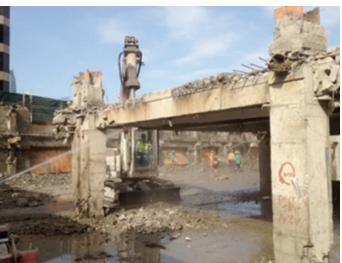
the asbestos materials. These materials will be removed with a combination of equipment, including specialized ultra high pressure water blasting devices and custom built negative air machines 20 times the industry standard.
