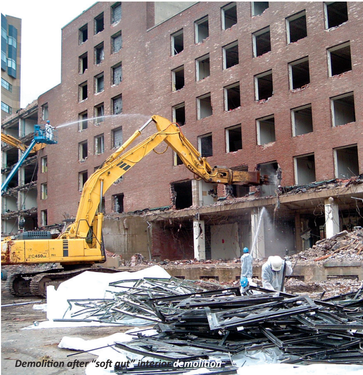
Structural demolition with LVI's high reach equipment
