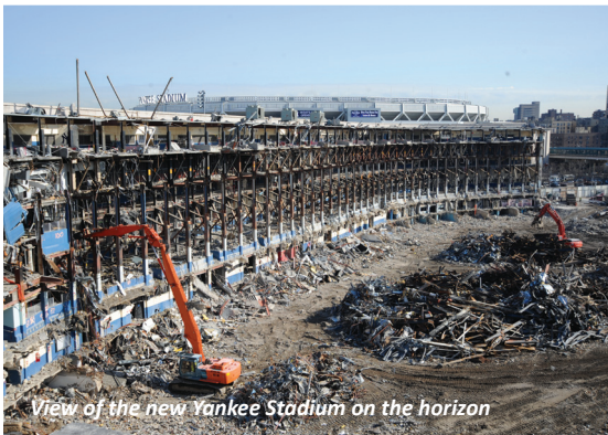
Demolition sequence of one seating section
