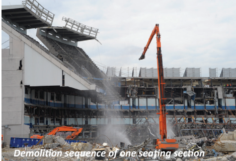
Demolition sequence of one seating section
