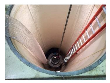
The TRIGA reactor assembly was located in a below-ground 20 foot deep steel reactor pool/tank structure with only vertical access to the core. The reactor assembly contained a graphite-reflected fixed core constructed of aluminum resting on a platform that raises the lower edge of the assembly about 2 feet above the tank floor.
