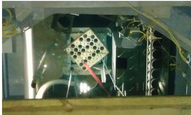
Grid plate unbolted from support stand and ready for packing
