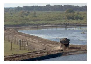
Our general scope of work includes: Clearing and grubbing, Gopher Tortoise relocation, Turbidity monitoring, Access road construction, Construction of a temporary culvert crossing, Fence installation, Excavation - Oxbow excavation/dredging involving 640,000 cubic yards through wetlands in order to construct 28,000 feet of new oxbows. In addition a spoil mound was degrading and used to backfill the C-38 canal and degrading and transportation of 850,000 cubic yards of material.
