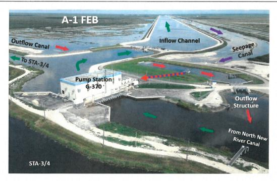
The A-1 FEB design further reduced operational and construction costs by utilizing solar-powered slide gates for the A-1 FEB discharge structures (10 Structures) that are located between the FEB and STA-3/4. These structures allow for the gravity discharge from the FEB to STA-3/4 reducing required pumping and at the same time eliminated the need of roughly seven miles of overhead power lines.
